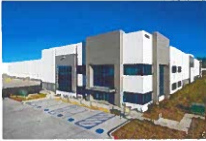
Typical Building Design with Concrete Wall Panels
